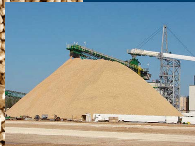
Foto: Green Circle Bio Energy
